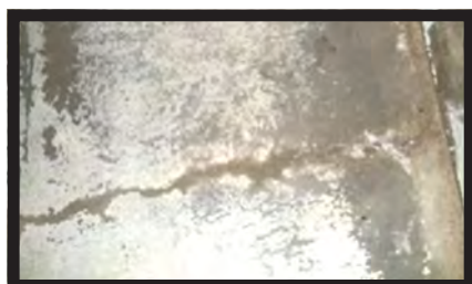
Figure 2 - Failure of Chemical Resistant Paint
