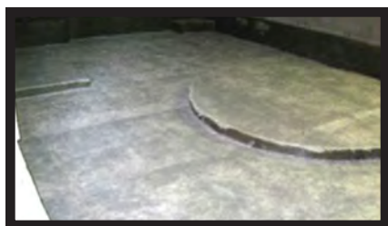
Figure 3 - Installation of Fiberglass Matting
